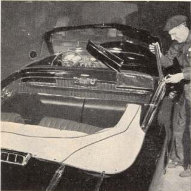
Pillar support for convertible's top folds sideways into partition and then is covered by hinged cap. Convertible is only one of the 10 cars without an extra radio for rear-seat passengers.
